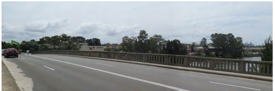
View 1 Existing - View from Canal Road bridge, looking North towards the city
