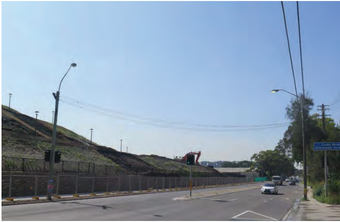
View 4 Existing - View from Canal Road, looking South-East towards site
